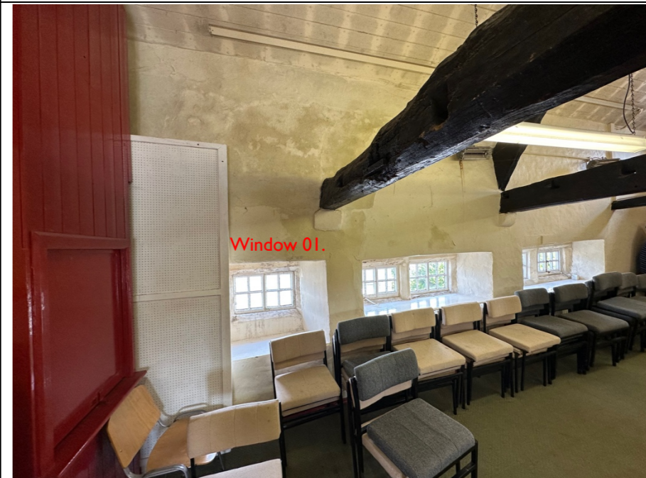
063 – View of the principal front elevation to the traditionally constructed Listed building. There is extensive discolouration and staining to the internal plastered wall finishes.
