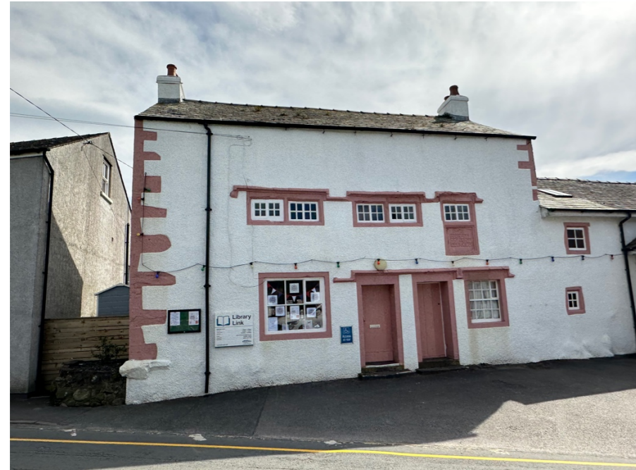
017 - General elevation of the traditional older building, all under a dual pitched natural slate roof covering, small timber framed windows, rendered walls and painted stone detailing. North West orientation.
