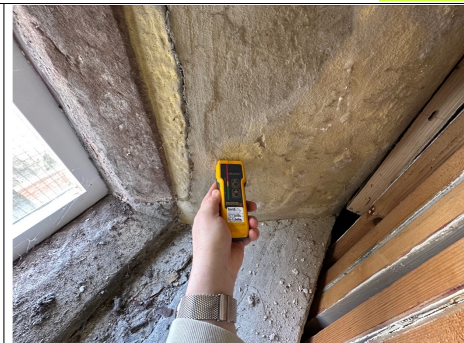
090 – Internal window reveal to the window opening identified in photo's 087 – 089.
