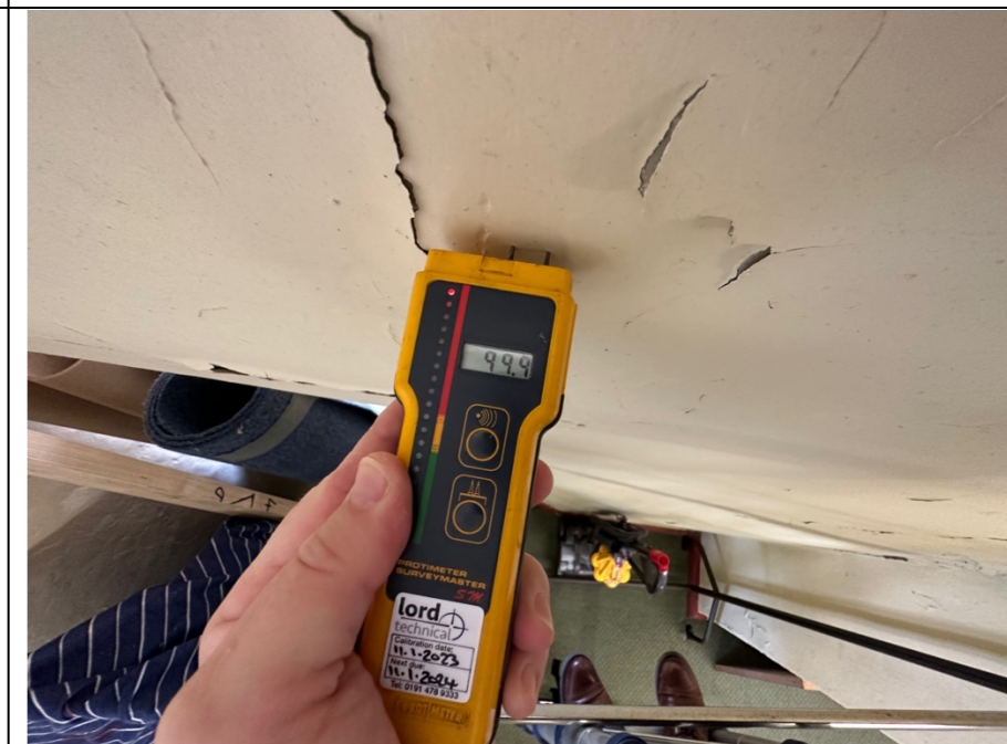
075 – Mid-level wall panel between the two windows identified in photo 074.
