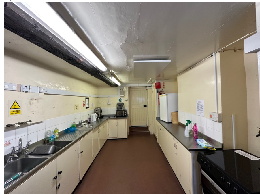
031 – Internal image of the kitchen area within the traditional Listed building, looking back toward the rear corridor which provides access to the Library area, toilets and the main hall.
