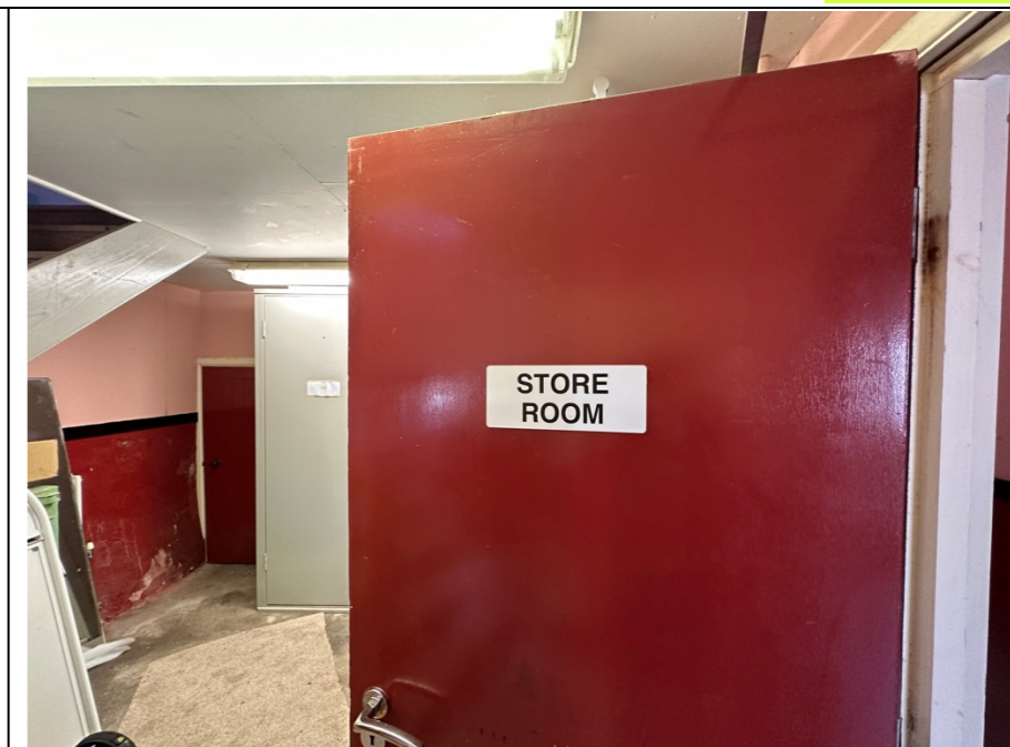
042 – General view of the ground floor store room area within the traditionally constructed Listed structure. For purposes of orientation the ground floor kitchen is to the left of this room, when viewed from this position.
