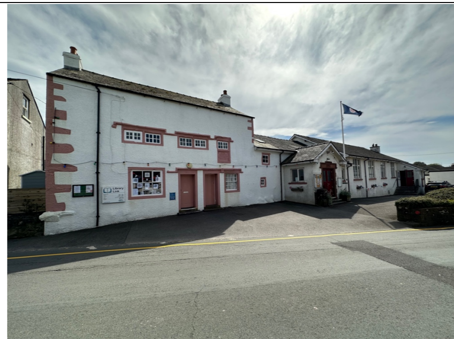
002 – General elevation of the traditional older building, all under a dual pitched natural slate roof covering, small timber framed windows, rendered walls and painted stone detailing. North West orientation.
