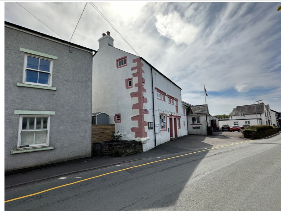
027 – General view of the building from the North East and looking onto the gable end wall.
