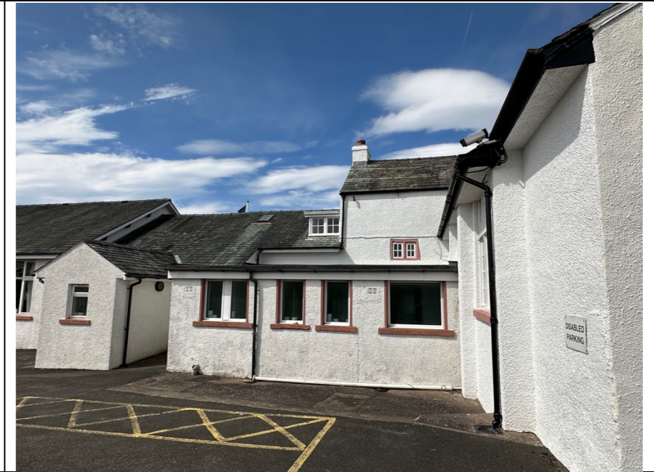
093 – General external view of the rear toilet extensions.
