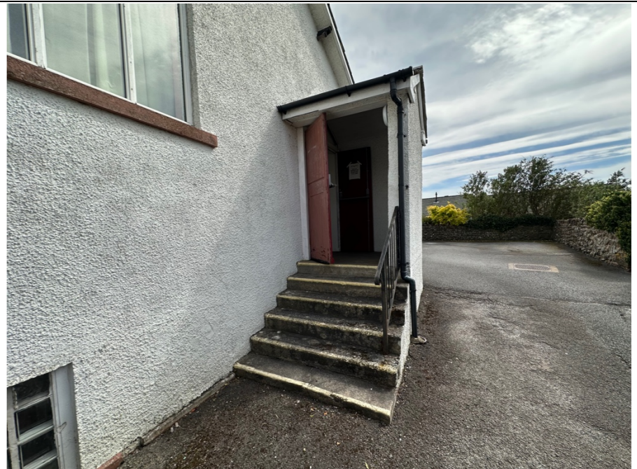
108 – General external elevation of the rear entrance / exit lobby.
