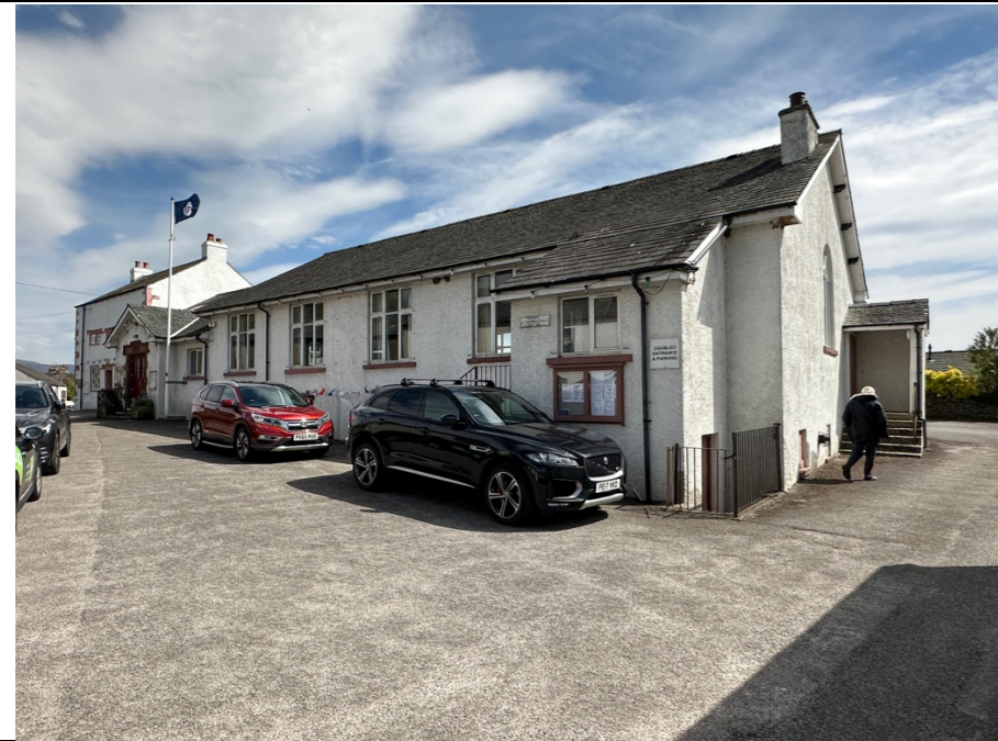
091 – General external elevation looking toward the North East across the front elevation of the Hall extension with the traditional building in the background.
