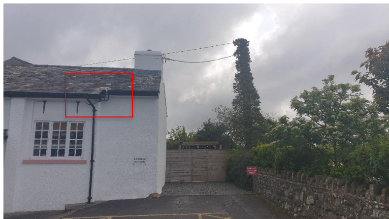
Location of existing camera
