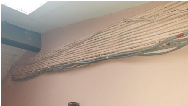
Poorly fixed and protected cabling
