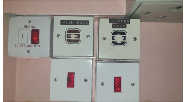
Heating extension timers
