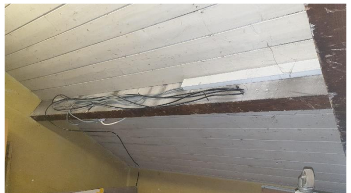
Poorly fixed and protected cabling
