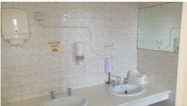
Instantaneous water heater - Female WC
