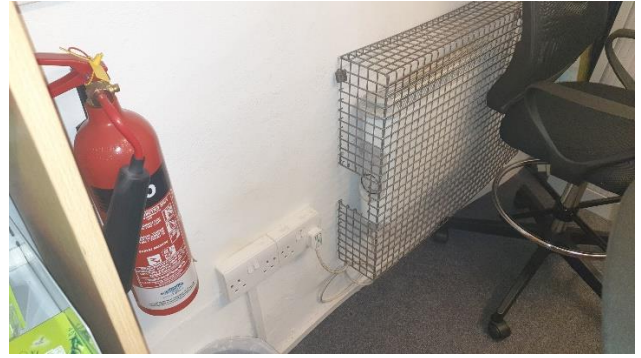
Electric panel heater
