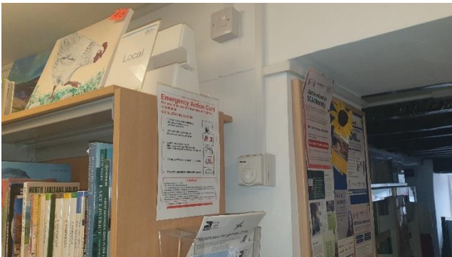
Radiant panel heater thermostat
