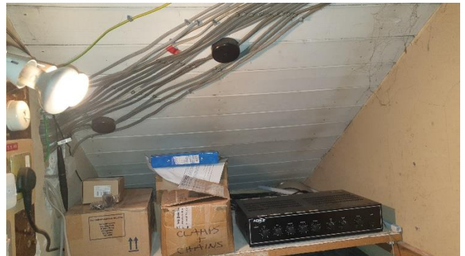
Poorly fixed and protected cabling
