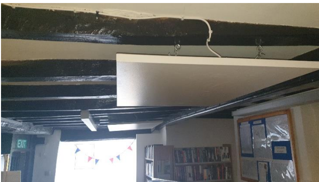
Electric radiant panel heater
