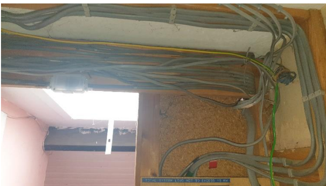
Poorly fixed and protected cabling
